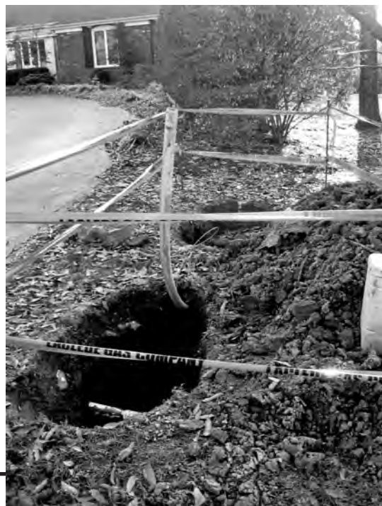
Gas line installation.
